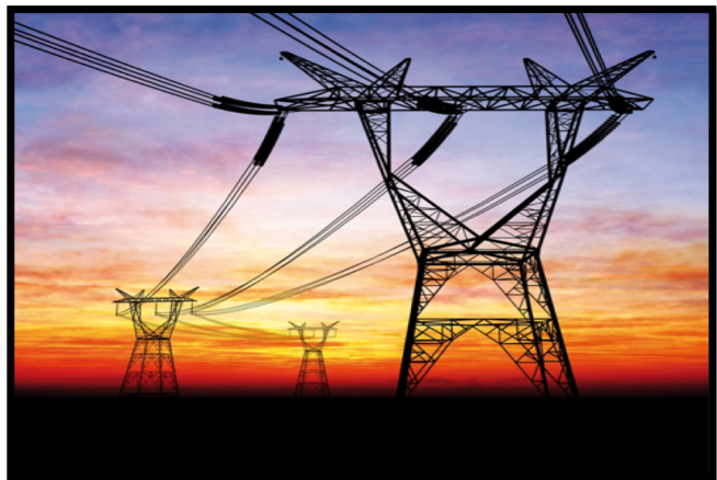
Electric Power Grid
